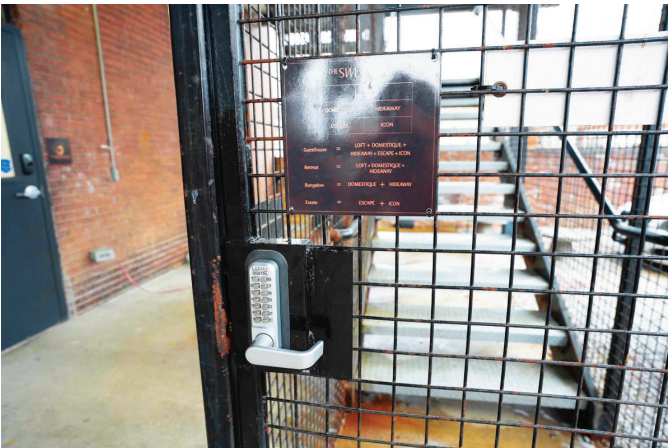
(View of exterior metal staircase)
